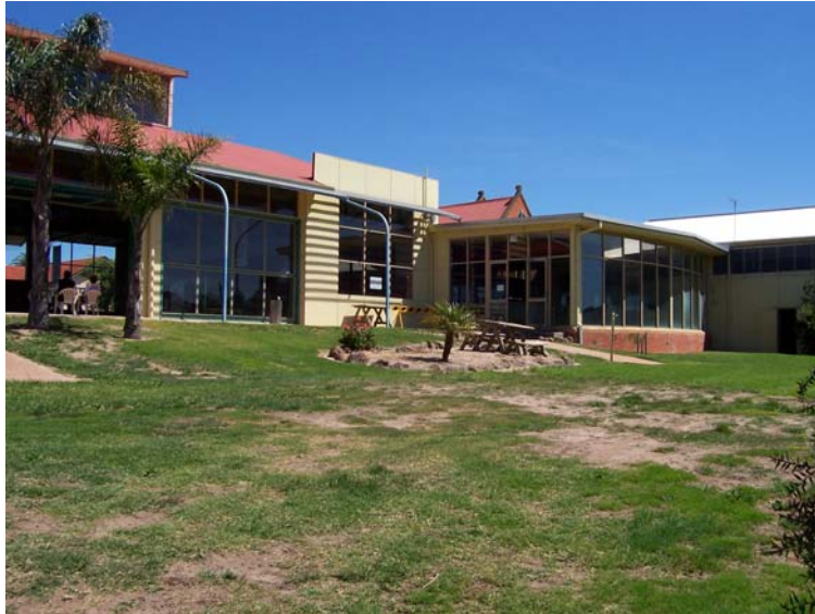
The Ararat Rural City Recreation and Aquatic Centre showing the only space available for further development unless existing buildings are demolished. This space has some potential for actions which do not use all the open area.
