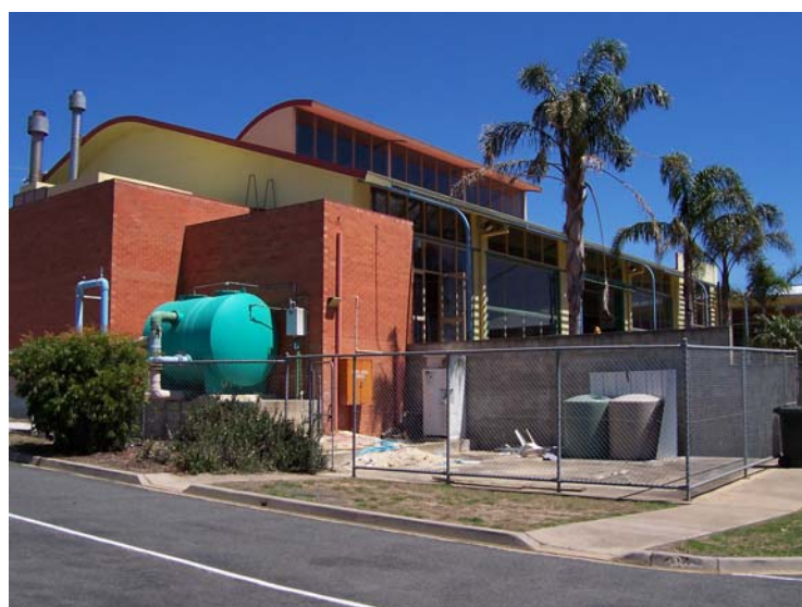
The indoor pool hall at Ararat Rural City Recreation and Aquatic Centre. Site constraints have meant that the facility plant room extends onto the nature strip of the adjoining street (foreground).
