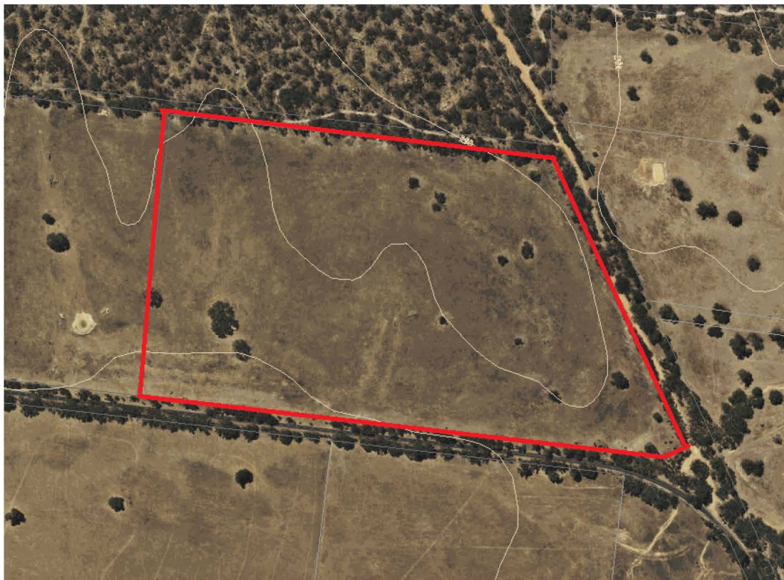
FIGURE 3 EXISTING CONDITIONS AIR PHOTO
