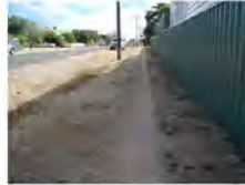
3 Lack of formal footpaths / unsealed footpaths
