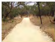
4 Typical 2m wide unsealed shared path
