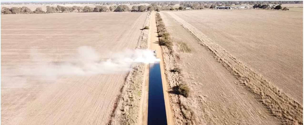
Image: New road seal applied to Andrews Lane. June 2024.
