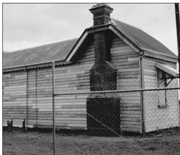
Most Heritage Places are able to be repaired: Pirron Yallock Railway Station before (top) and after repair (below)
