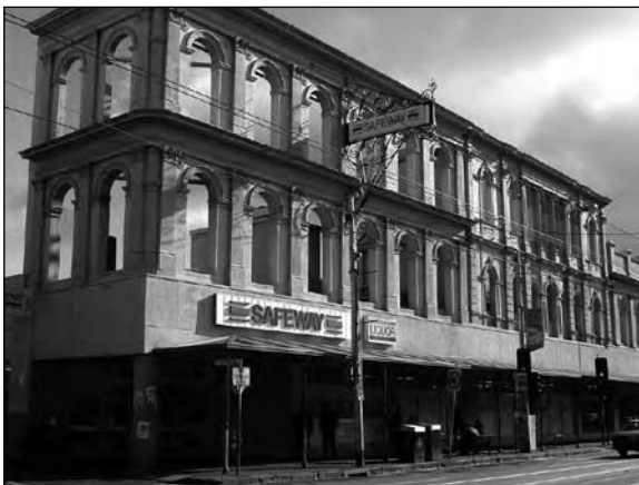
Facadism resulting from inadequate fabric retention
