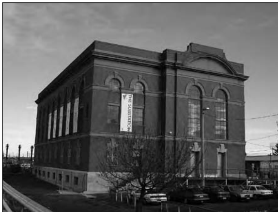
Adaptive reuse of an industrial Heritage Place: the former Newport Railway Electricity Substation undergoing conversion to a community arts centre
